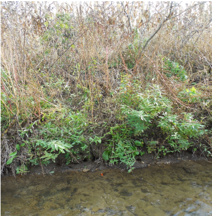
Photo S. Ave.-2: Left Bank (E)
