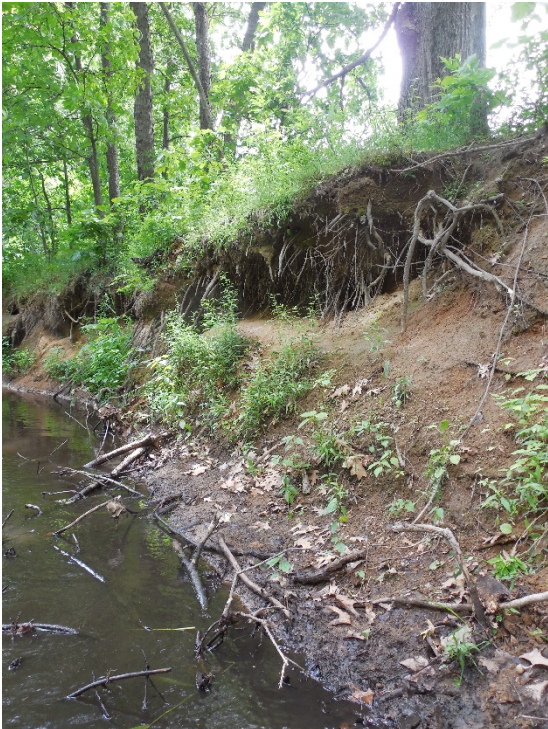
Photos Y Ave.-2: Right bank (W)
