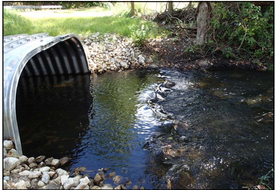
Figure 4. Rock ramp structure below the new culvert on Pigeon Creek.
