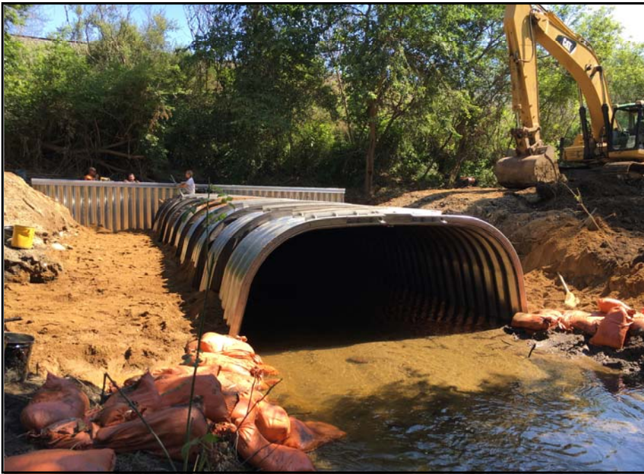
Figure 3. New culvert installation on Pigeon Creek, Calhoun County, Michigan.
