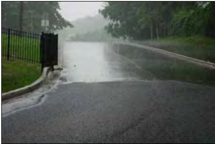
Figure 50 – LID Example: Porous Pavement (foreground) Willard Park, Battle Creek, Michigan
